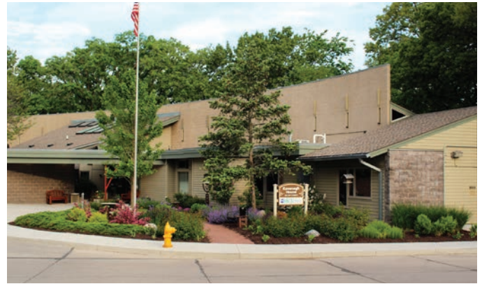
Kavanagh House on 56th Street in Des Moines opened in 1993. It was one of Iowa’s first residential hospice facilities and serves up to 15 individuals in private rooms.
